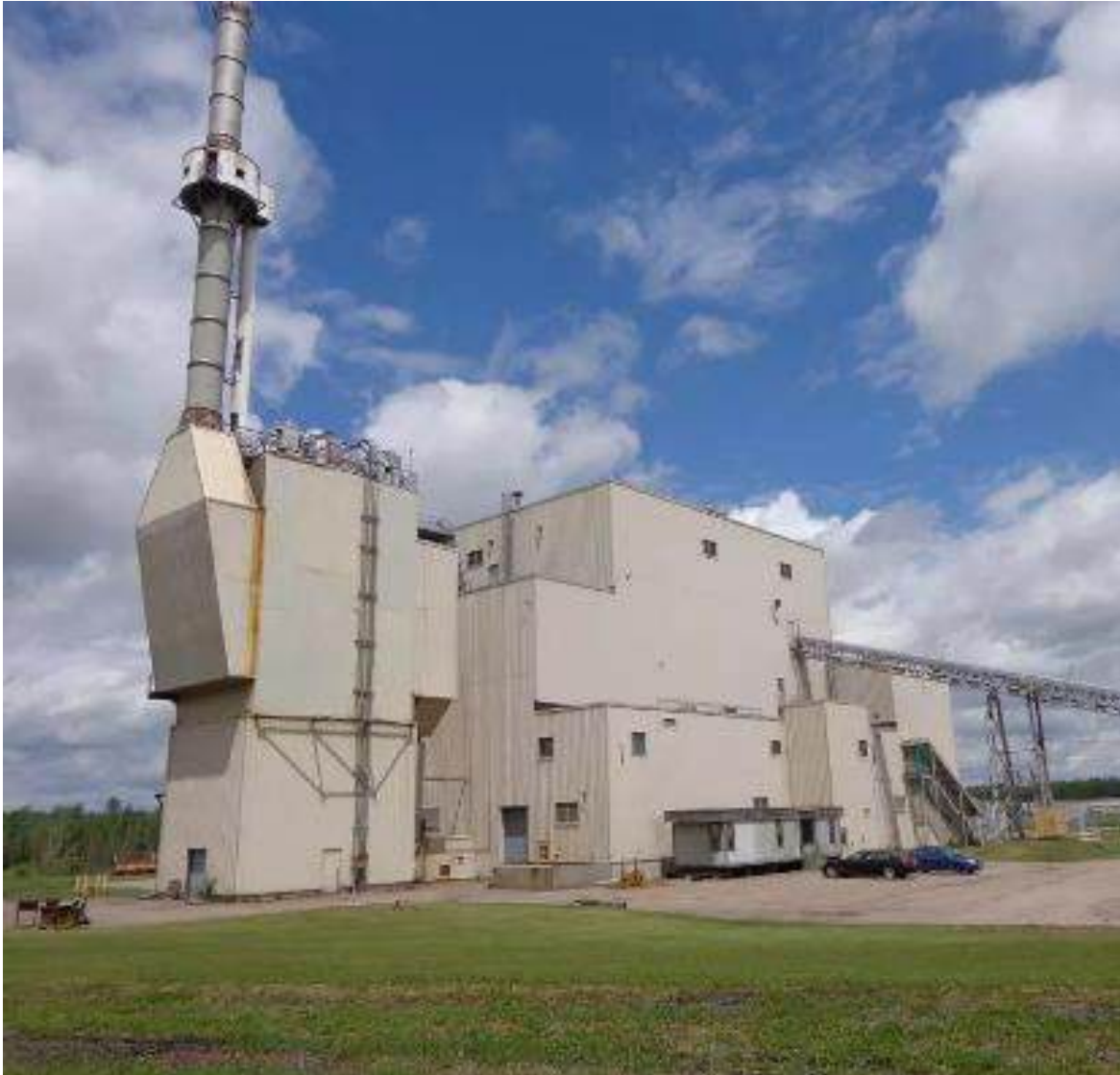
Picture of the biomass power plant
