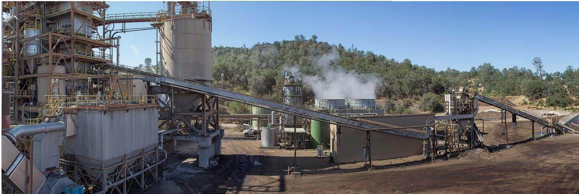
Picture of the Buena Vista, CA, biomass power plant
