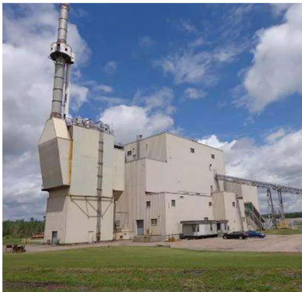
Picture of the biomass power plant
