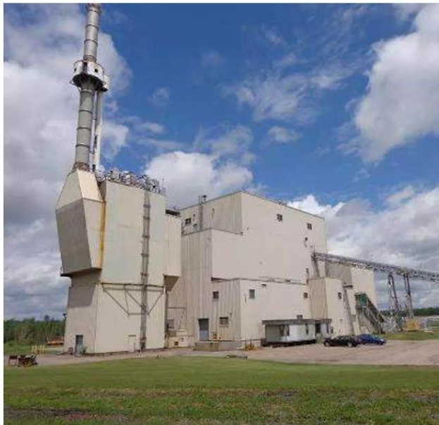
Picture of the biomass power plant
